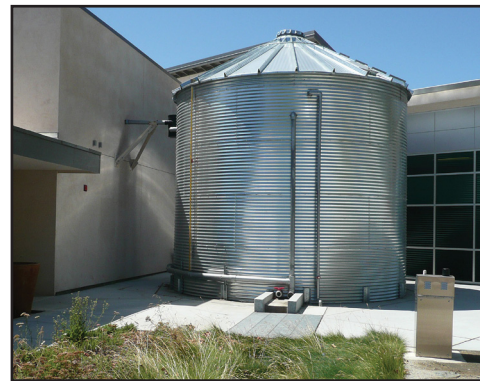
A 20,000-gallon cistern at New Technology High School in Napa.
